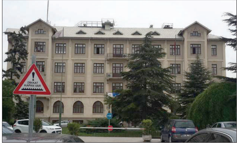
Figure 16B. Building and Lodgings of State Railways Administration. Architect: A. Kemalettin Bey. Date: 1925-1928. Photograph by: D. Avcı Hosanlı, 2015.
