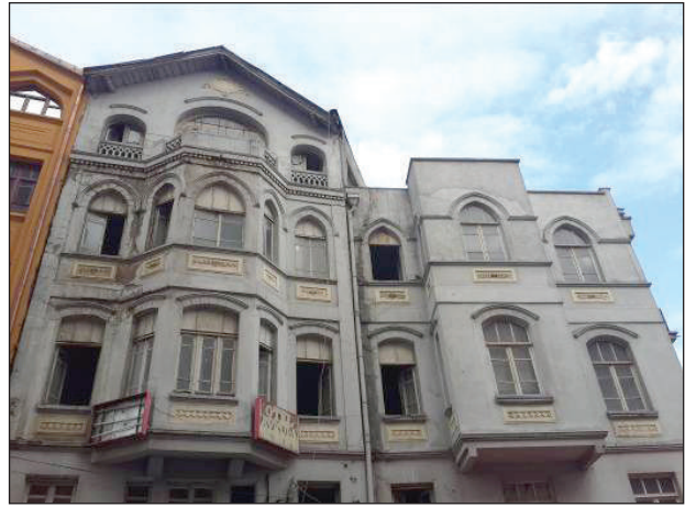
Figure 2B. Avrupa Hotel and its addition. Date: 1916/1917-1920s.
