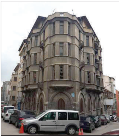
Figure 7A. Erzurumlu Nafiz Bey Apartment (Işıklar Street, No: 27). Date: 1922.
