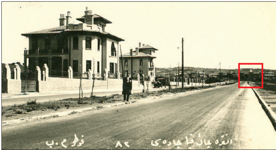
Figure 20A. Fevzi Paşa Mansion (Yenişehir). Architect: Arif Hikmet Koyunoğlu. Date: before 1928. Source: VEKAM Library and Archive, Inventory no: 2480.
