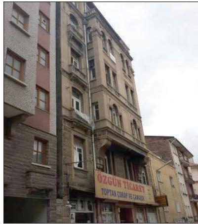
Figure 7B. An apartment (Işıklar Street, No: 22). Date: before 1927.
