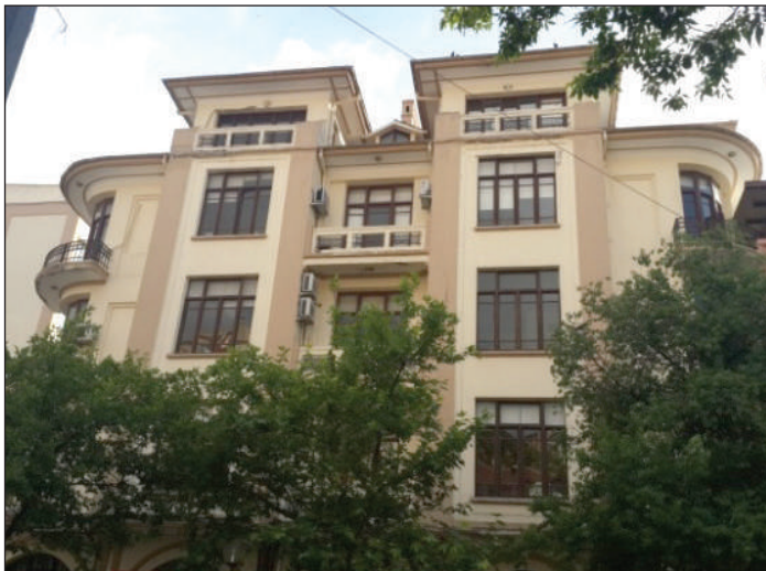
Figure 12A. Children's Protection Agency and its rental apartment (Çocuk Sarayı (Anafartalar) Street). Architect: Arif Hikmet Koyunoğlu. Date: 1926. Photograph by: D. Avcı Hosanlı, 2018.
